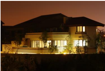
Fig. 7, Extended Terraces linking outside spaces with the reception and guest house, Author, 2017.
