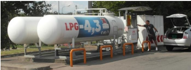
Figure 1. LPG pressure vessels in petrol stations: above: unprotected pressure vessels, below: pressure vessels protected with anti-ram fence (author's photos)
