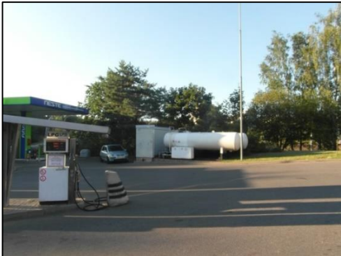
Figure 1. LPG pressure vessels in petrol stations: above: unprotected pressure vessels, below: pressure vessels protected with anti-ram fence (author's photos)
