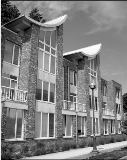
Figure 3.16. Externally reclaimed bricks, C.K Choi Building
